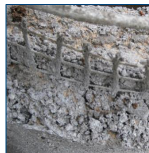
Integration in Abwasserrohr
